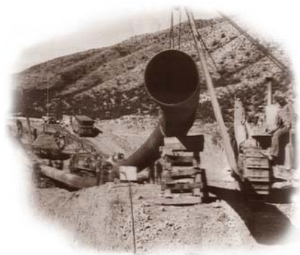
SARAKHS - NEKA 800 KM, 30"/36" DIA GAS TRANSMISSION PIPELINE
